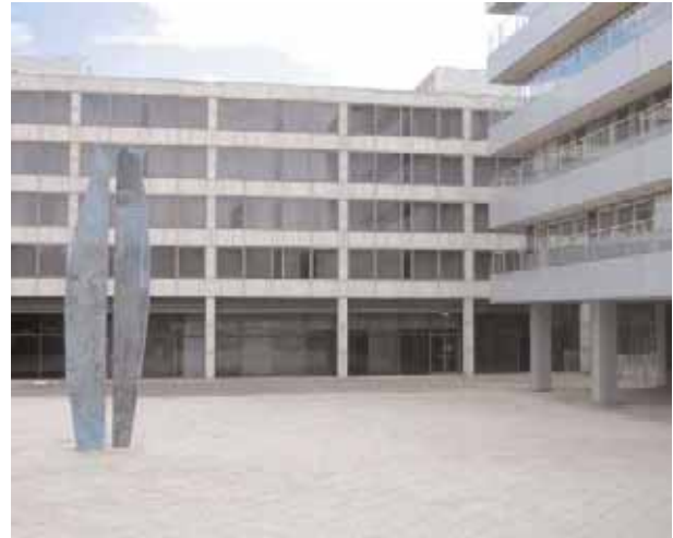
Blank elevations fronting an empty space - a 'no go' place in Milton Keynes
