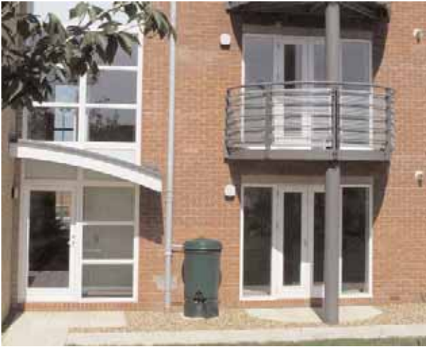
Rainwater harvesting in Milton Keynes
