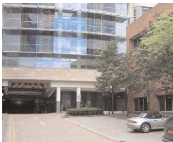
Servicing for a major retail scheme accommodated within this building in central Milton Keynes
