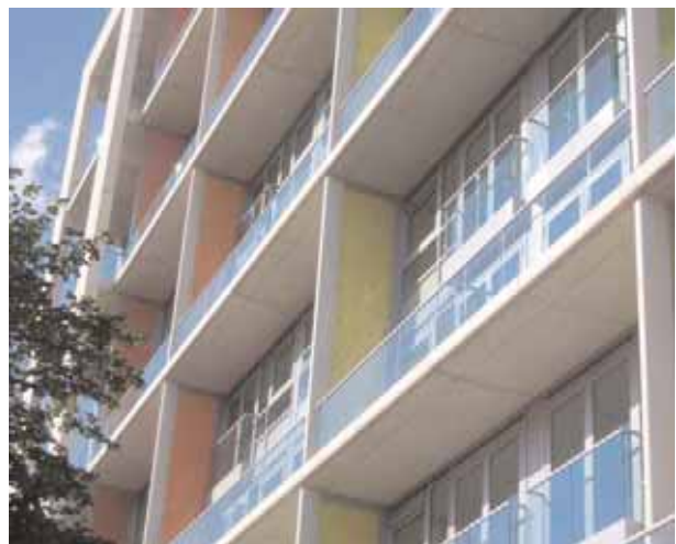
Good sized balconies provide private amenity space and enliven this building's appearance
