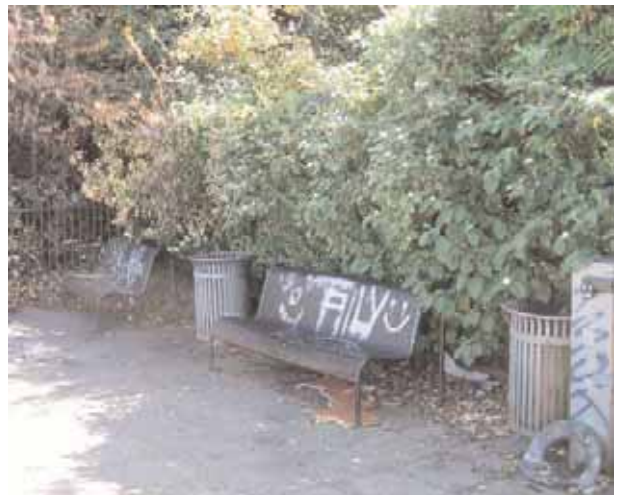
Minimal overlooking of this cliff top space in has resulted in neglect and vandalism
