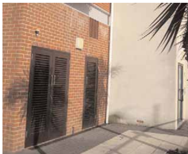
Bin storage and services are integrated into the design of this building at Gunwharf Quays in Portsmouth
