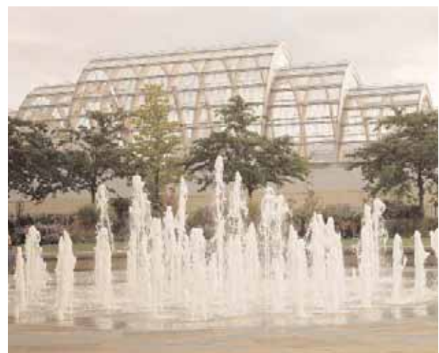
Sheffield Winter Gardens provides a glazed backdrop to a new square
