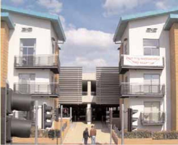
A multi - storey car park is 'wrapped' by apartments in Brierley Hill in the West Midlands
