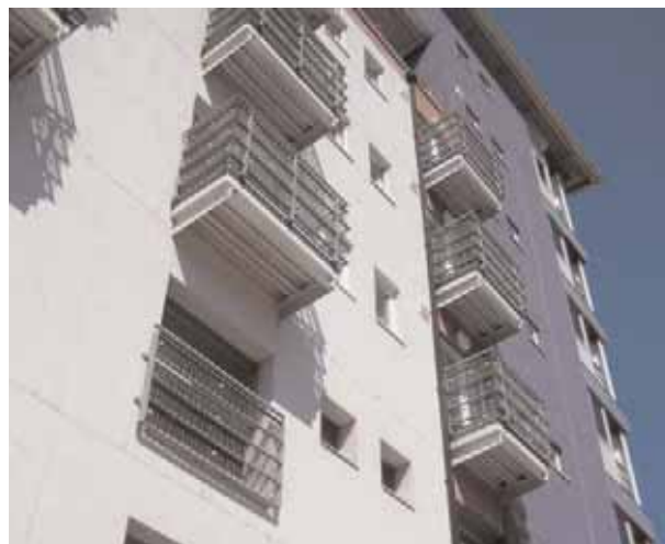
Well scaled and detailed development at St Peter's riverside
