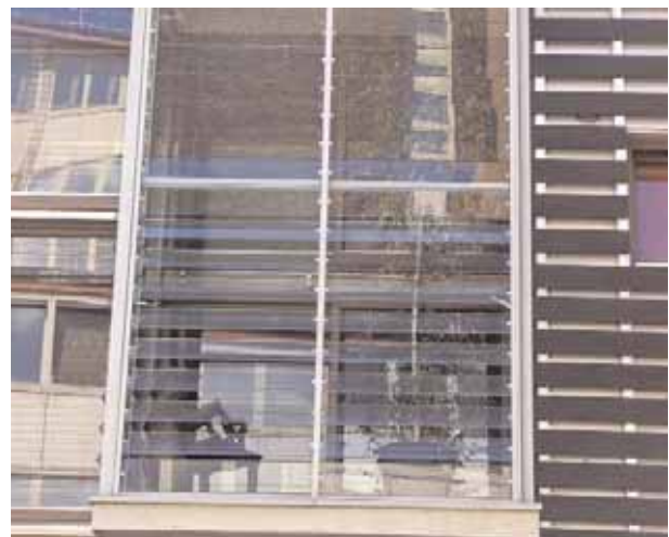
A carefully detailed middle section adds variety to this residential scheme in London
