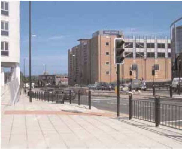
A new surface crossing at West Wear Street replaces an underpass
