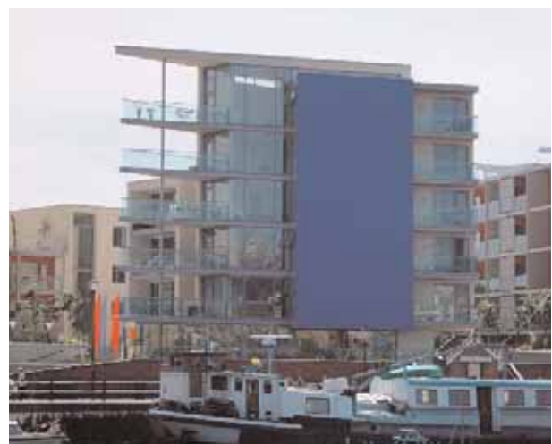
Well detailed balconies overlook the waterfront at Bristol
