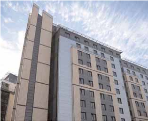
A service tower at this hotel in Nottingham creates a landmark at a site close to the station
