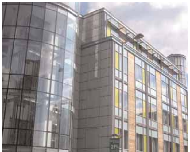
Gateway development adjoining a major junction in Nottingham fronts and contains the space
