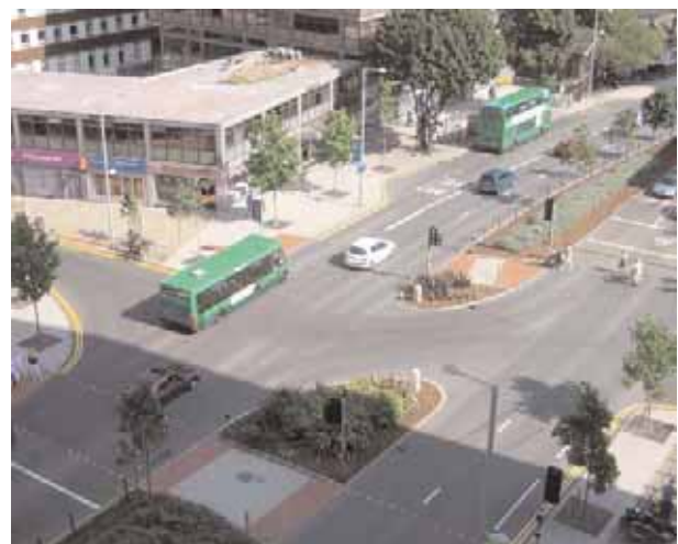
Here, a roundabout has been replaced with a simple junction with direct crossing points. . . . .
