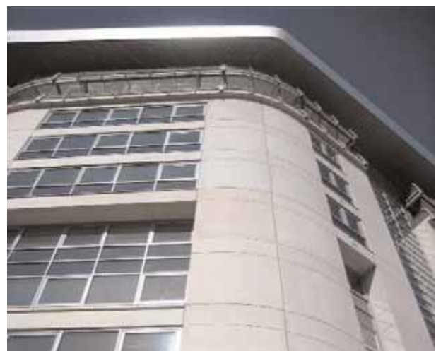
Echo 24 provides a landmark adjoining 'City Gate'
