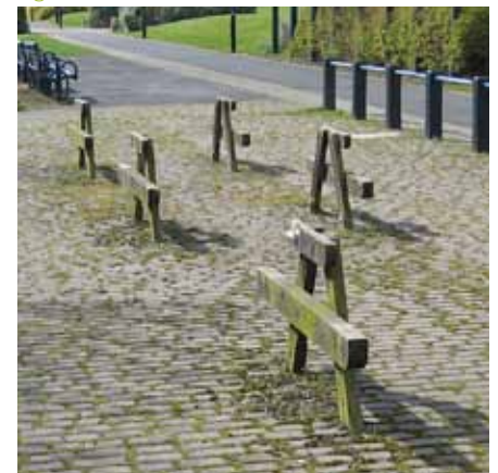
Signs of recent vandalism
