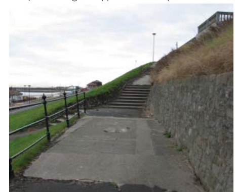
Footpath linking the upper and lower promenades
