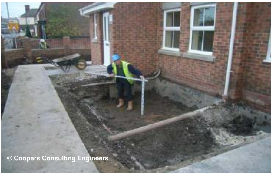
© Coopers Consulting Engineers
