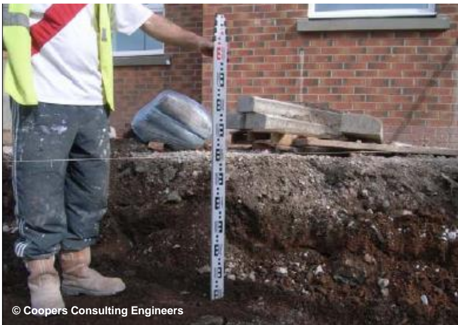
© Coopers Consulting Engineers
