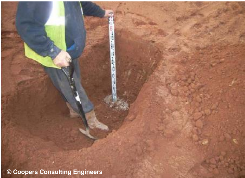
© Coopers Consulting Engineers
