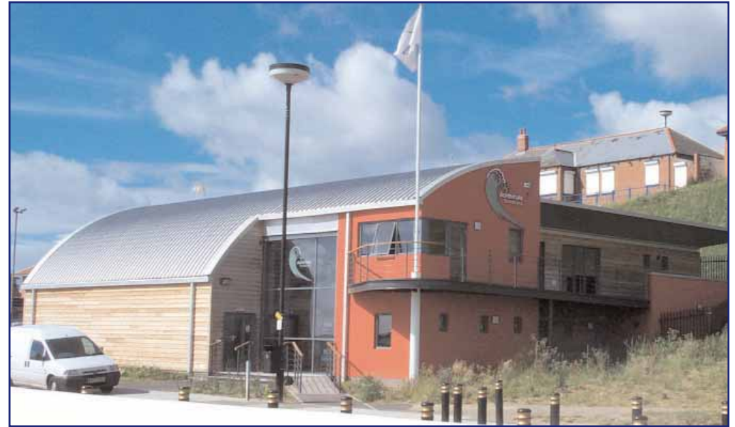
This development on Marine Walk responds well to the surrounding landscape and displays a quite innovative design that is appropriate for its beach front location.
