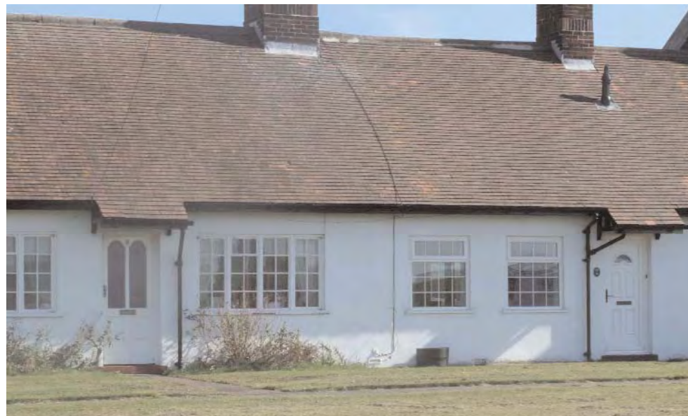
Changes to the window openings and windows to accommodate replacement PVC units have insensitively altered the historic form of the property to the right; the property to the left has retained its original appearance.
