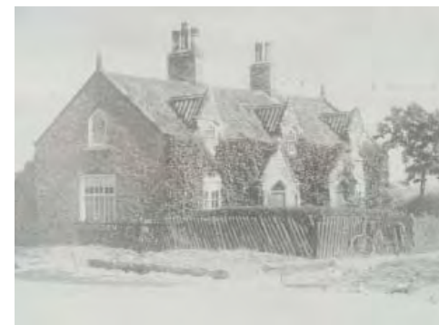
Cottages at north end Source: Reeder (1992)
