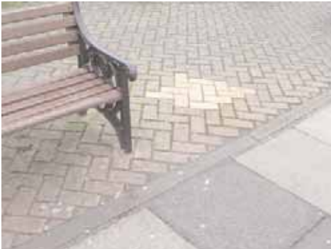
Above left: Poor mix and quality of surface materials, poorly repaired and with chewing gum stuck on flags. Above right: 'barrel' planters have been installed to add colour and interest to the street scene.
