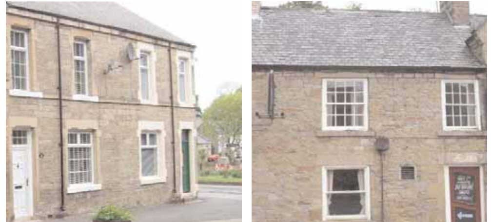
Non-traditional uPVC windows appear incongruous on this historic stone property (above left), particularly when compared to the timber sliding sashes on the pub (above right).
