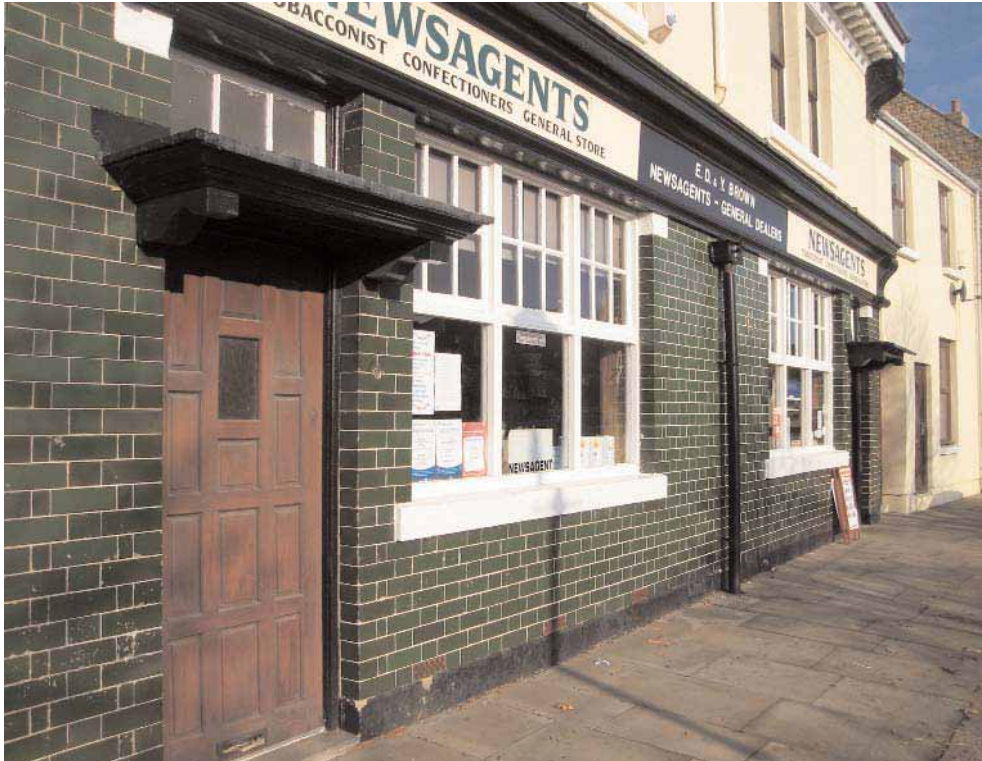
The fascia signage on the Newsagents is a good example of the use of simple and discreet lettering.
