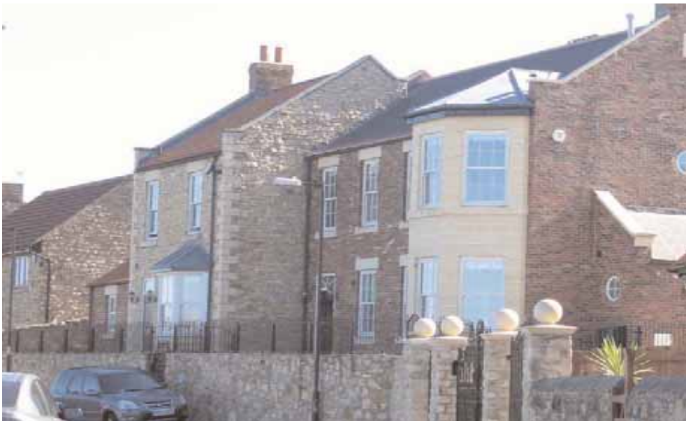
These recently built properties respect and reinforce the building line, form and materials of historic properties along North Street. The use of uPVC windows does however detract from the buildings and general street scene.
