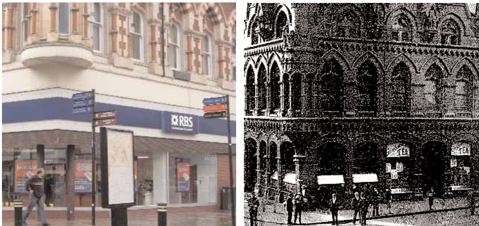
Above left: an unsympathetic modern shopfront on a landmark building, compared with the original frontage in the late 1800s, right.
