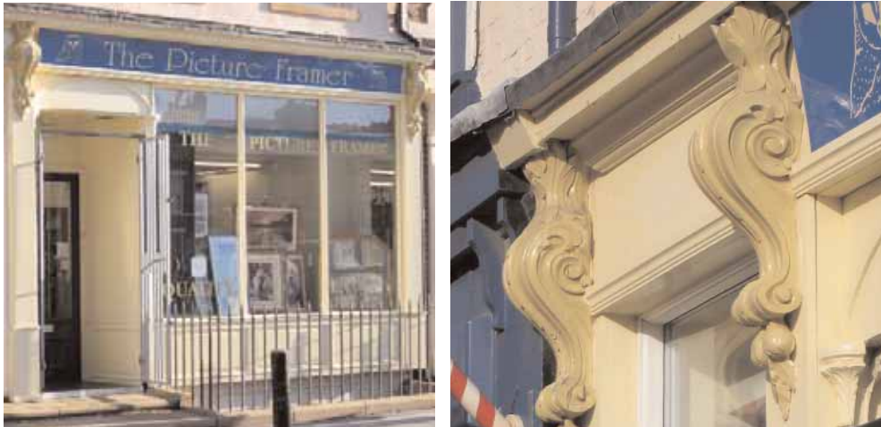
Above: a traditional shop front on Norfolk Street, complete with decorative consoles
