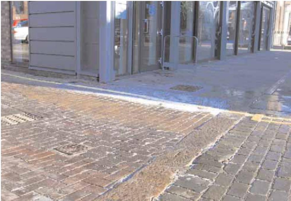
Complementary mix of traditional materials around thePlace, some historic and some newly laid.
