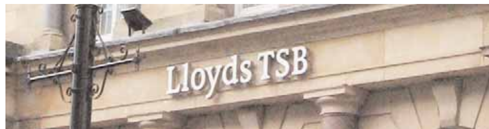
Above: freestanding individual lettering on a Listed sandstone building minimises the impact of the commercial signage on this historic property. Although the signage is not in the Bank's usual style and is devoid of corporate colours and logos, it is nonetheless distinctive and easily recognisable, demonstrating that a sensitive conservation-led approach to signage does not jeopardise the advertising potential of a business.
