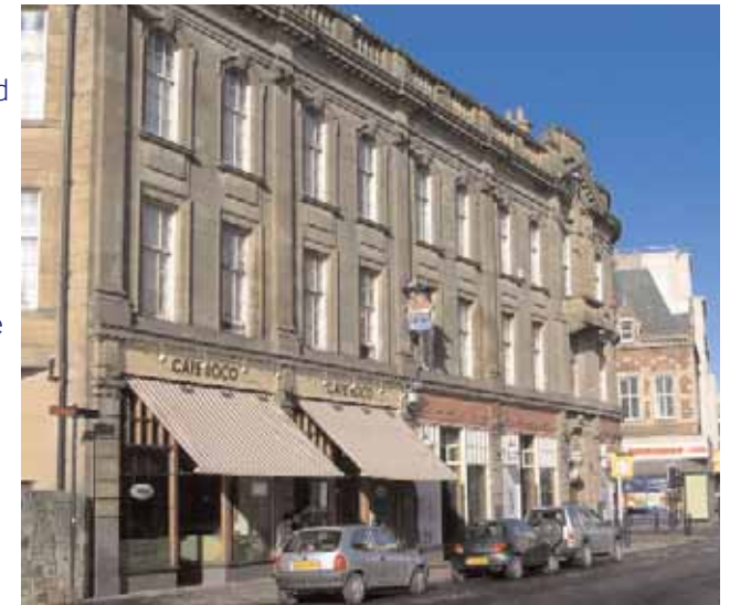
Above: recently restored shop front of Cafe Roco on Burdon House - a fine example of a traditional frontage.
