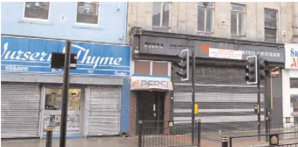
Above: the deadening effect of external roller shutters, which are discouraged throughout the city but are particularly inappropriate in a conservation area setting.
