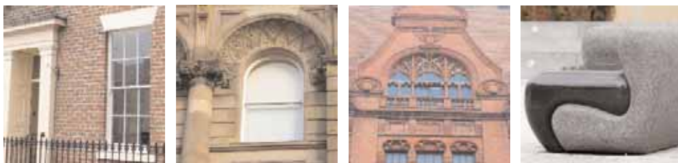
Above: Garden wall bond brick terrace with timber detailing; carved sandstone and ashlar on the former Hutchinson's building; terracotta on Sydenham House; polished granite street furniture in Sunnyside Gardens.
