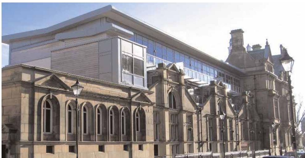
Contemporary extension to the old Post Office, enabling this landmark listed building to be brought back into beneficial use as apartments.
