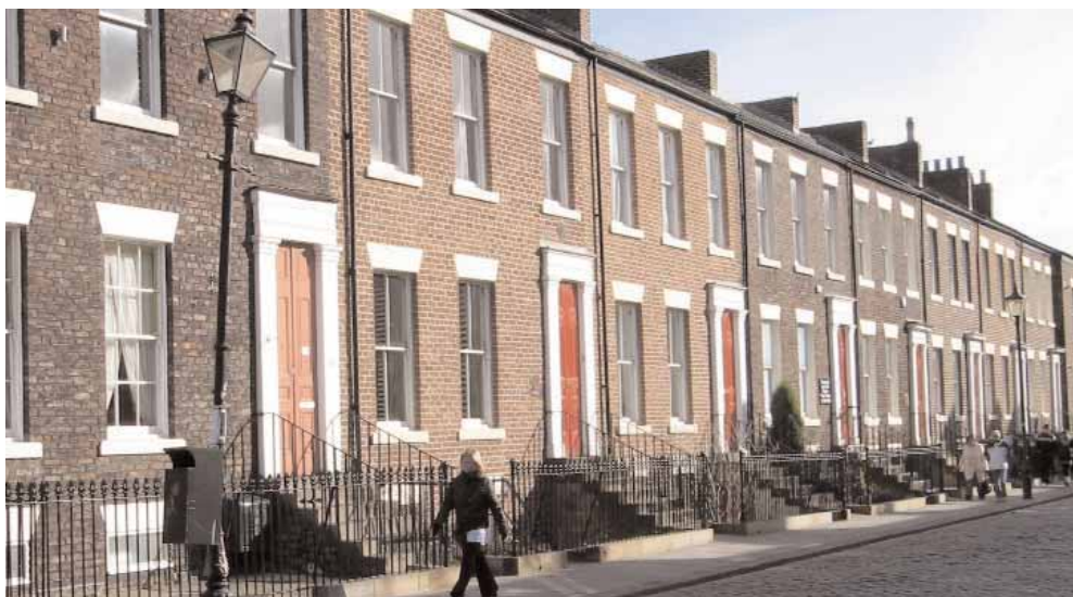
A uniform colour scheme in action, above, on Foyle Street. These properties were restored to their original splendour by Gentoo, with assistance from the Sunnyside THI; the scheme adheres to the established colour scheme for the terrace
