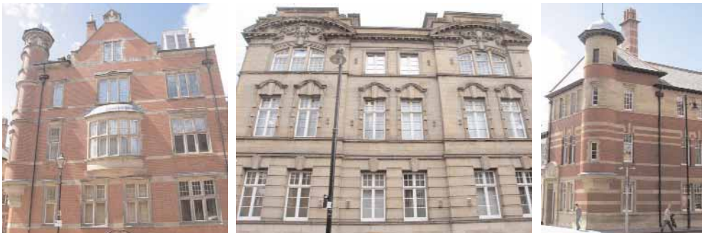
Maritime Buildings; River Wear Commissioners' Building; Sunnyside Chambers
