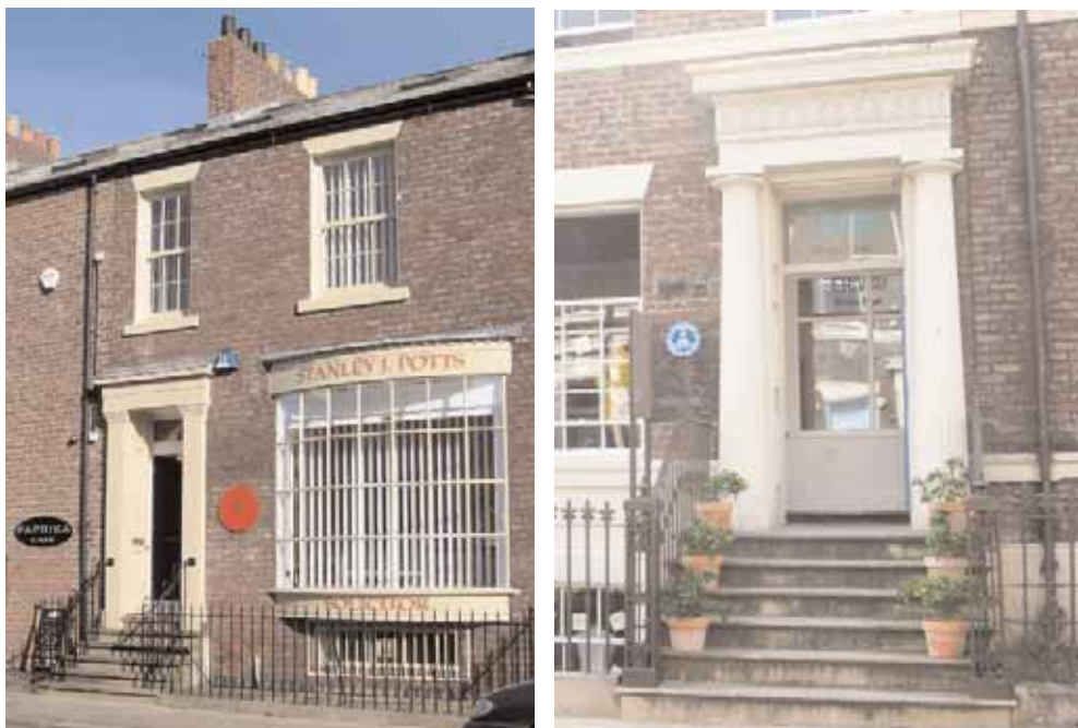
Above left: despite a large shop window, inserted many years ago, this property on Frederick Street has largely retained its domestic appearance: such interventions will not, however, be allowed in future. Above right: this shop on John Street retains all of its domestic characteristics, with subtle signage.
