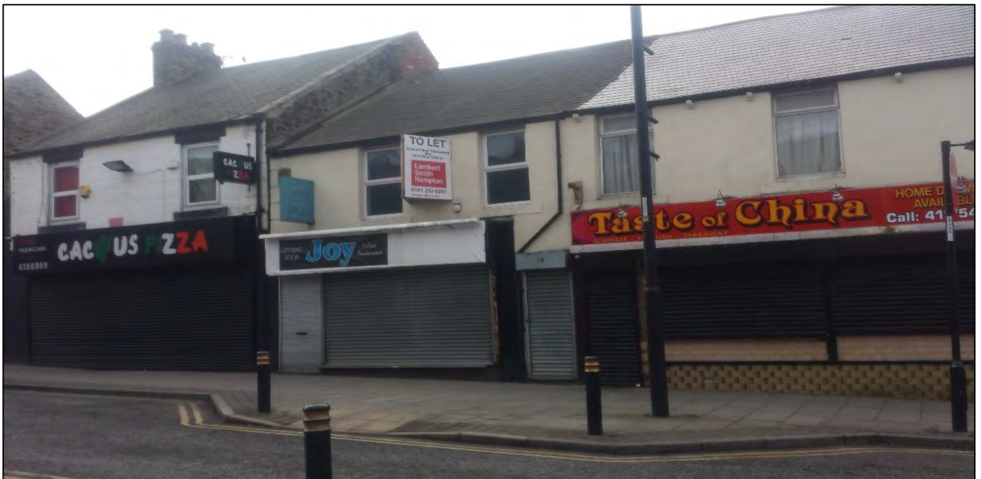
Photo 1 – Two Takeaway units and a vacant unit clustered together along Speculation Place
