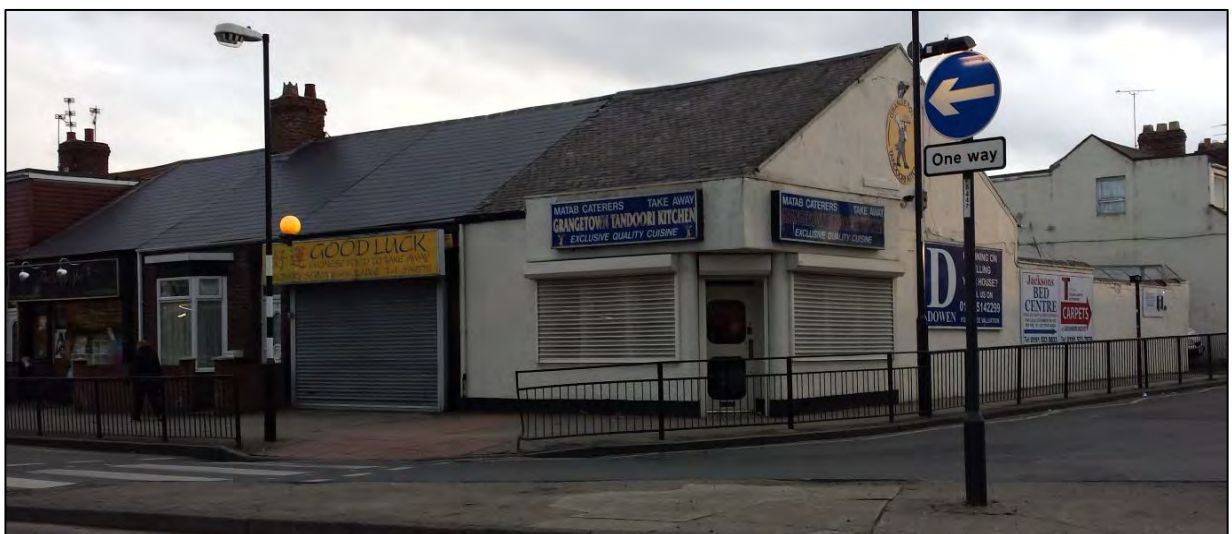
Photo 5: Shows the set of two adjoining takeaway units within Grangetown Local Centre
