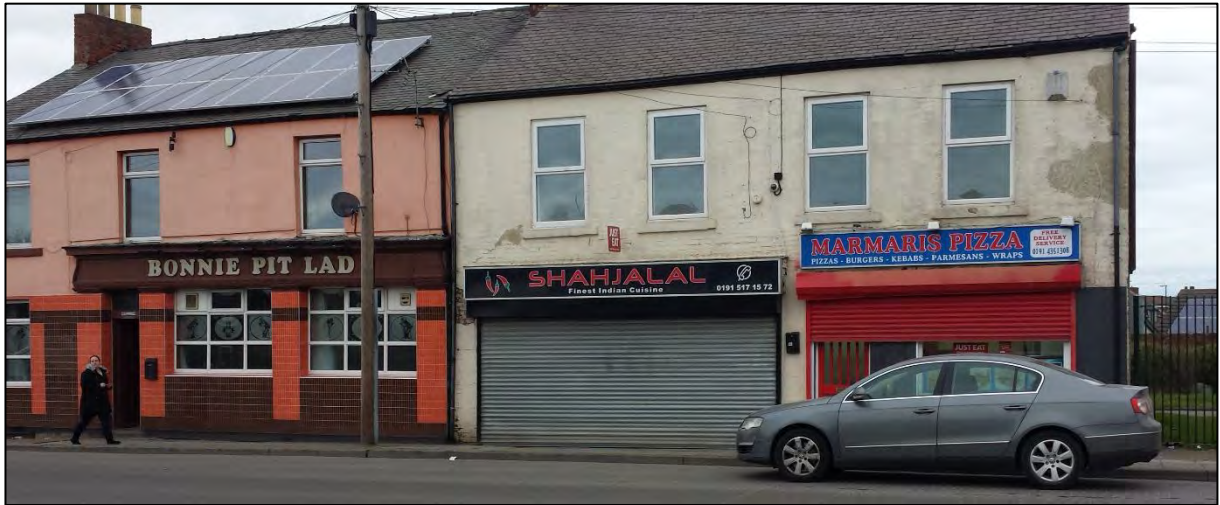
Photo 12: Shows the two adjoining takeaway units within Easington Lane Local Centre
