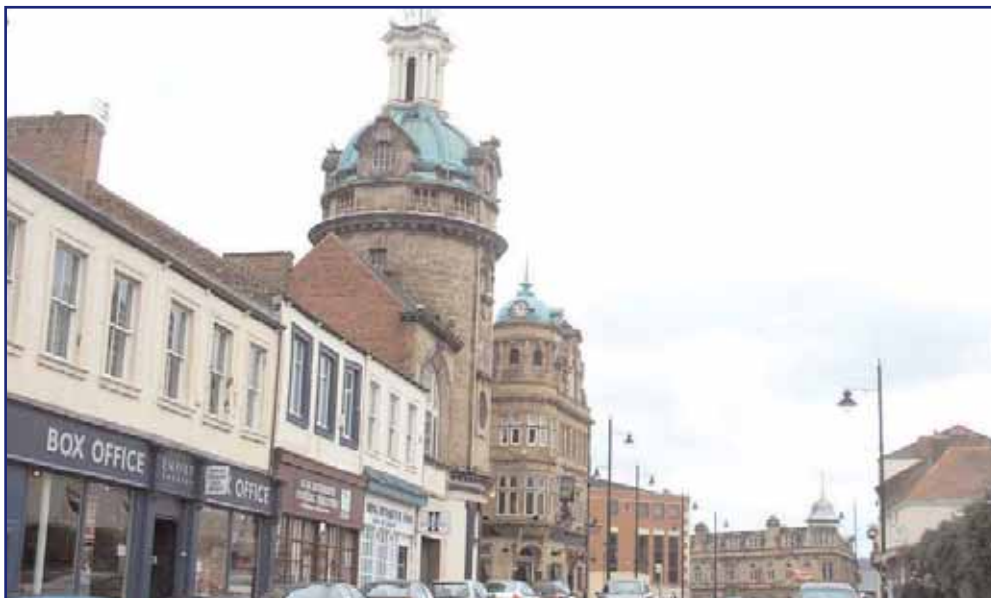
The variety building forms, styles and materials adds significantly to Bishopwearmouth's character.
