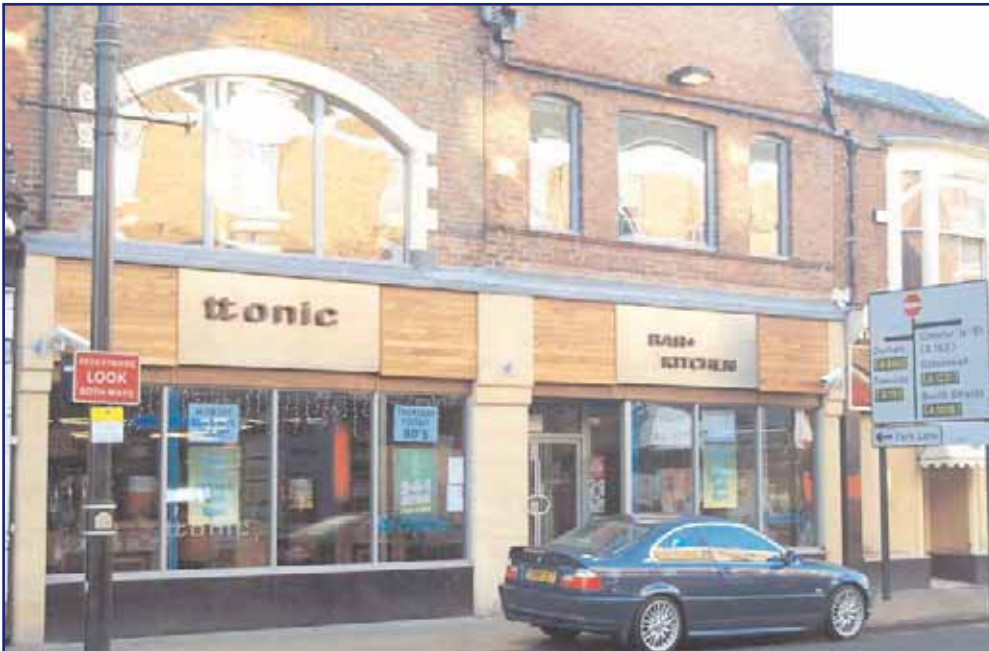
The shop front above successfully mixes traditional and contemporary materials in a simple yet high quality modern design to provide an attractive frontage that relates to the upper floor.
