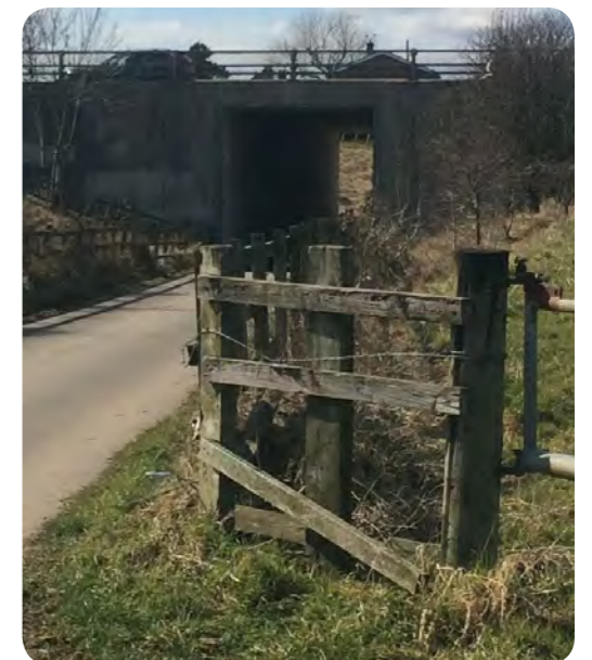
Underpass to Wood House Farm
