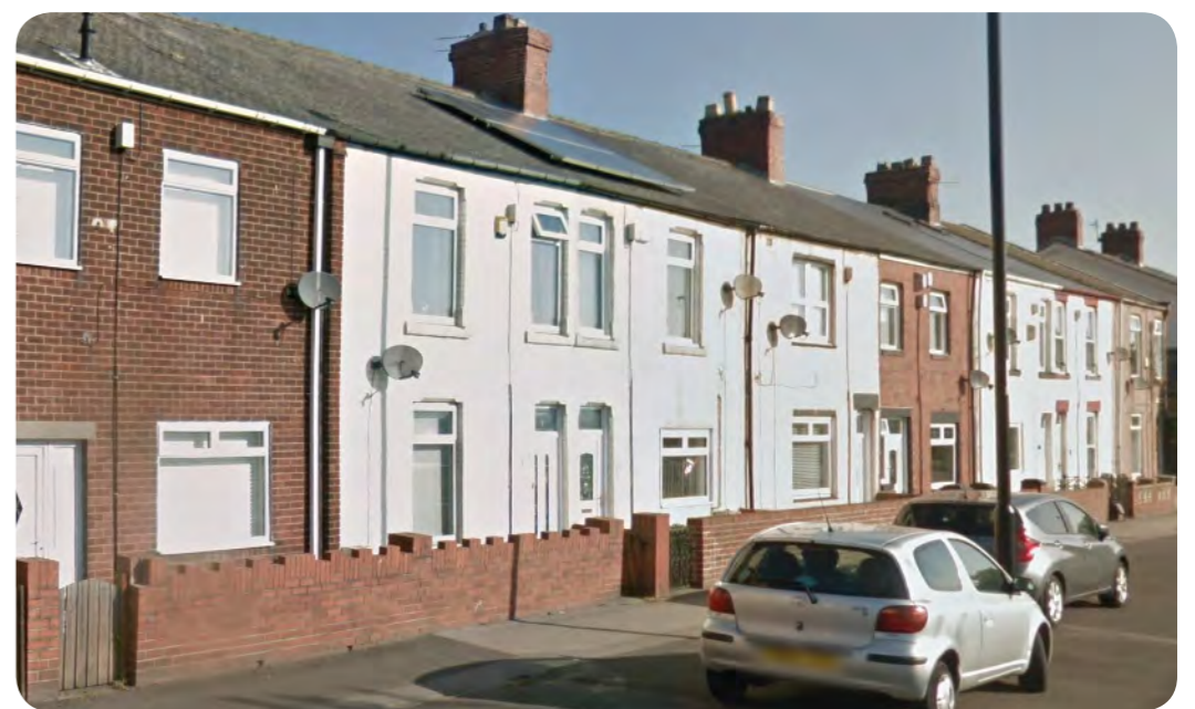
Existing housing on Chester Road
