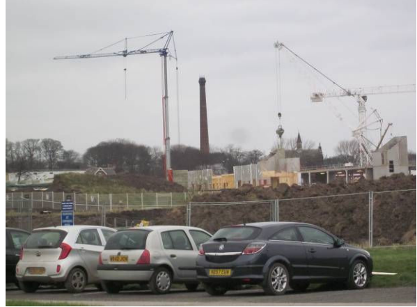
P26: Hospital redevelopment works
