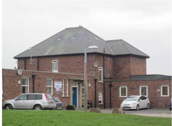
P24: Hospital buildings
