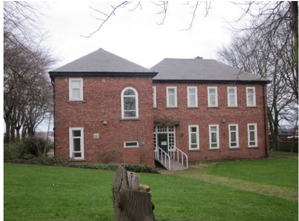
P22: Hospital buildings
