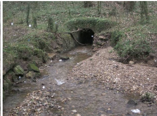
P30: Culvert in Cherry Knowle Dene
