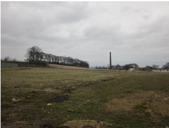
P21: Heras fencing and hospital demolition
