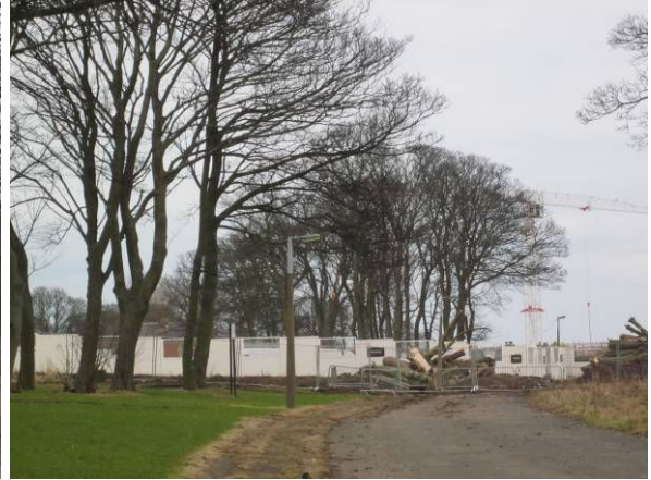
P20: Hospital construction & clearance works
