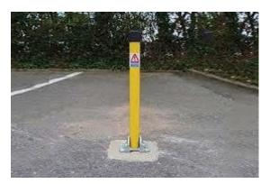
The bollards are to be surface mounted steel and complete with a bracket for the Customers own padlock similar to the one shown in the above photo. The post is to be square or round 100mm x 100mm with an overall height of 750mm finished polyester powder coated yellow. It is to be surface mounted onto a 300mm square concrete foundation which is to be 300mm deep and fixed to the concrete with concrete fixings. The bollards are to be of a good quality, grade and weight.
