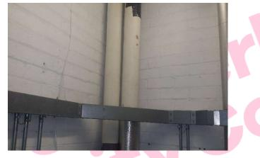
The pipe lagging in Rm 043/Boiler Room does not contain asbestos.
