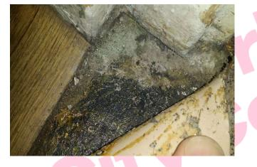
The remnant adhesive backing to floor in Rm 020/Cleaners Store contains asbestos.
