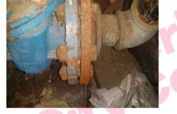
The gasket to pipework in Rm 043a/Gas Meter Room does not contain asbestos.
