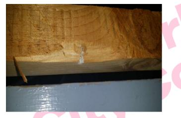
The residue to beams and joists in Rm 040/Classroom – void above contains asbestos.
