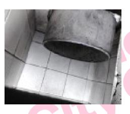
The flue pipe in the cavity wall seen through the grilles in the Boiler Room is presumed to contain asbestos.
