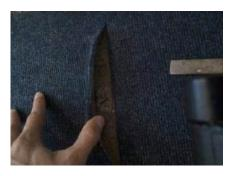
The adhesive to the concrete floor beneath the modern lino to the electronic engineers (Room 24) does not contain asbestos.
