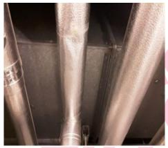
The mastic to the vessel in the Plant Room (Area 2) does not contain asbestos.
