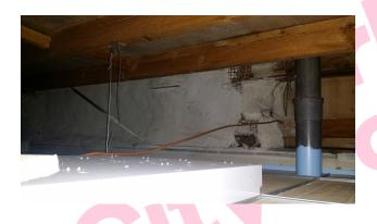
The firebreak & associated debris in 027/boys wc -void above does not contain asbestos.
