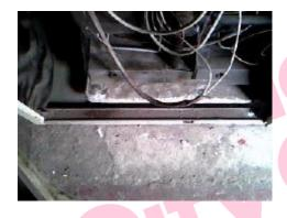
The insulating board plinth to boiler 1 in Room 1 Boiler House does not contain asbestos.
