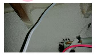
The firebreak & associated debris in 01/entrance lobbyvoid above does not contain asbestos.
