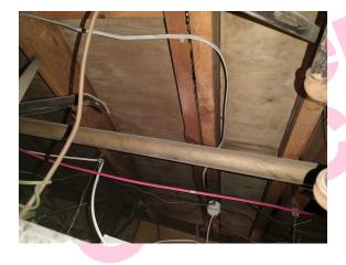
The roof adhesive residue to joists in Kitchen void above/ 0/20 does not contain asbestos.
