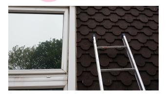
The brown sealant to clay tile wall cladding (External) does not contain asbestos.
