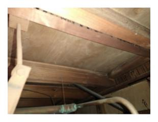
The roof adhesive residue to joists in Kitchen locker room void above/ 0/21 does not contain asbestos.
