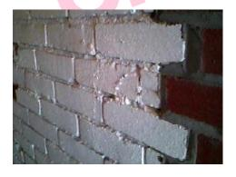
The debris to wall in Room 1 Boiler House does not contain asbestos.
