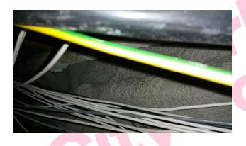
The firebreak & associated debris in 024/girls wc -void above does not contain asbestos.
