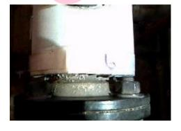
The debris around gasket in Room 1 Boiler House does not contain asbestos.
