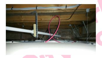
The firebreak & associated debris in 021/boys wc-void above does not contain asbestos.
