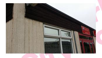
The render to walls & fascia (External) does not contain asbestos.
