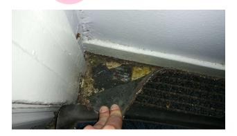
The subfloor covering in 022/corridor contains asbestos.
