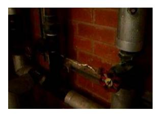
The debris to pipework in Boiler Room does not contain asbestos.
