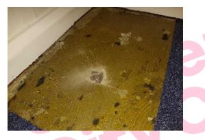
The brown adhesive residue below modern screed (Adhesive) (Area 4/Year 4 Classroom) does not contain asbestos.
