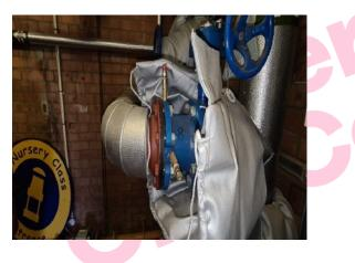
The Pipework flange gaskets (Boiler Room) does not contain asbestos.
