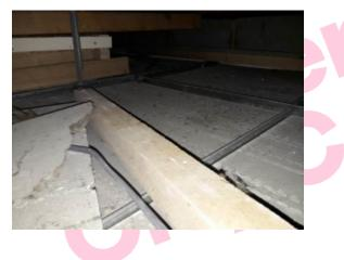
The debris to suspended ceiling (Pupils Toilet) does not contain asbestos.
