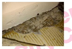
The brown adhesive residue below modern screed (Area 7/Lower KS2 Cloakroom) does not contain asbestos.
