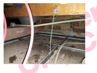
The debris to suspended ceiling (Medical Room 2) does not contain asbestos.
