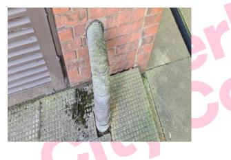
The Tape wrapping to gas inlet pipe (External) does not contain asbestos.
