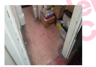
The floor screed (Cupboard G/003) does not contain asbestos.
