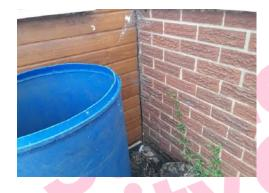
The expansion joint putty (Area 25/External) does not contain asbestos.
