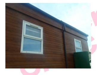
The window putty/seal to frame (External E/001) does not contain asbestos.
