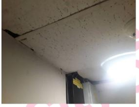
The wall lining in the electrical cupboard (G006) does not contain asbestos.
