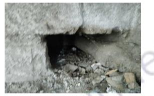
The damp proof course to walls (Bitumen) (Area:1 Garage) does not contain asbestos.
