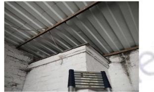
The roof - felt over WC and Lobby area ceiling (Bitumen) (Area:2 Workshop) does not contain asbestos.
