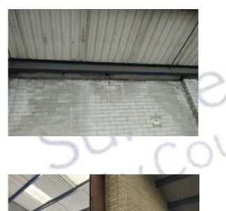
The rainwater goods – cement rainwater troughs (Cement) (Area:2 Garage 2) contain asbestos.
