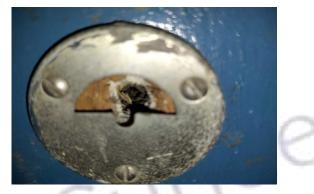
The door – panel within door (insulating board) (Area:5 Wash Area) contains asbestos.
