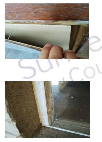
The door – insulating board firebreak panels within large central roller doors (insulating board) (Area:1 Garage) contains asbestos.
