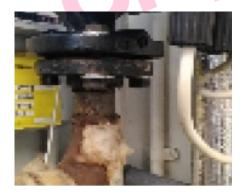
The gasket to pipework (Plant Roo/Room 002) does not contain asbestos.
