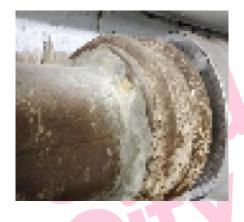
The packing to pipework (Boiler Room/Room 001) does not contain asbestos.
