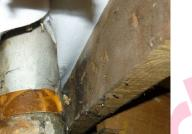
The coating to the elbow of the flue pipe in the loft space (Area L1/03) contains asbestos.
