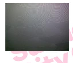
The coating to the ceiling in the stairs and landing (Rm 0/02) does not contain asbestos.
