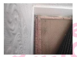
The bitumen adhesive to floor (Living Room) does contain asbestos.
