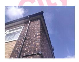
The Cement Soffits (External) are presumed to contain asbestos.
