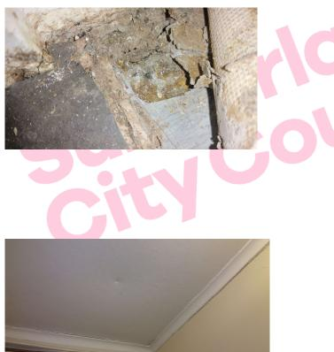
The remnant adhesive to concrete floor (below screed) in the WC lobby (Room 0/04) contains asbestos.
