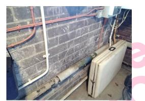
The Debris/Residue - to walls under window - Thermal Insulation Lagging in Boiler House/Changing Rooms G/004 Boiler Room does not contain asbestos.
