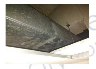
The mastic to the duct joints in the Office (Area 19) does contain asbestos.
