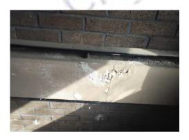
The horizontal boxing in the stairwell (Area 1) does not contain asbestos.
