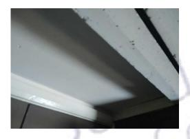
The ceiling in the stairwell (Area 1) does not contain asbestos.
