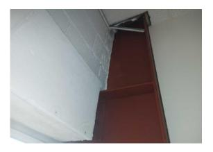
The boxing to RSJ's in the Office (Area 20) does not contain asbestos.
