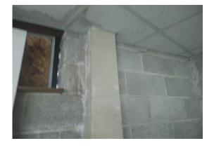
The boxing in the Observation Room (Area 16) does not contain asbestos.
