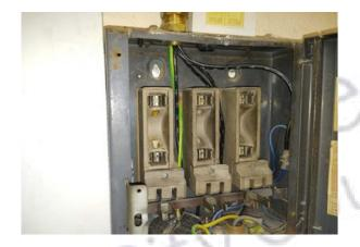
The mastic to screw holes on fuse carriers in the Office (Area 25) does contain asbestos.
