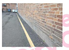
The damp proof course (bitumen) (Area: 06 building externals) does not contain asbestos.
