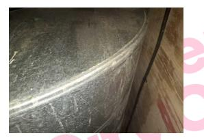
The ductwork joint mastic (Area: 05 boiler room) does not contain asbestos.
