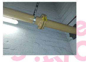
The pipe flange gasket (Area: 05A corridor) is presumed to contain asbestos.
