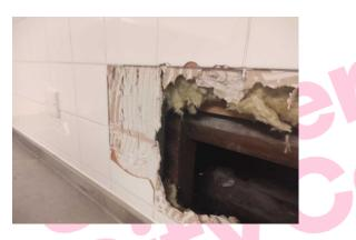
The walls (ceramic wall tiles adhesive) (Area: 3/42 kitchen) do not contain asbestos.
