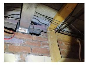
The cement shuttering within ceiling void (Area 80/WC accessible) is presumed to contain asbestos.
