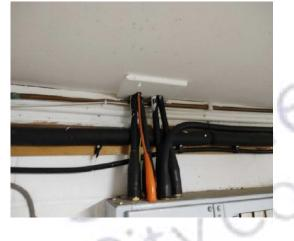
The infill panels to pipe penetration on ceiling (insulating board) in Area 20 – Cellar does not contain asbestos.
