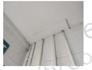
The infill panels to pipe penetration on ceiling (insulating board) in Area 24 – Garage Lobby does not contain asbestos.
