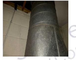
The mastic to ducting joints in Area 28 – Boiler Room does not contain asbestos.
