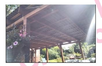
The roof – sheet cladding to the conservatory/sun room (External E/002) does not contain asbestos.
