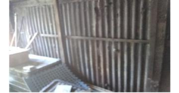
The wall sheet cladding to the garage (External E/003) does not contain asbestos.
