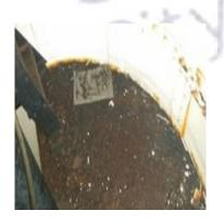
The top section of the metal staircase is severely corroded and is not safe to access.
