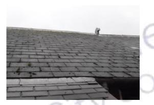
The roof tiles (External to roof /002) contain asbestos.
