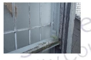
The putty to windows (External to roof /001) do not contain asbestos.
