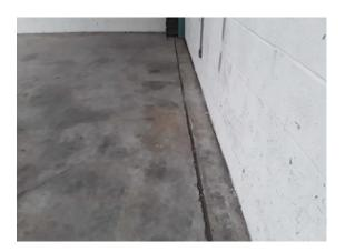
The expansion joints to floor (Area 1/Main factory floor) do not contain asbestos.
