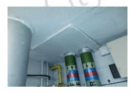
The ceiling panel to flue penetration in the Boiler Room (Area 001) does not contain asbestos.
