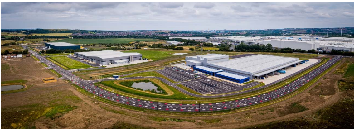
Figure 2.6 Photograph of the three industrial units looking eastwards
