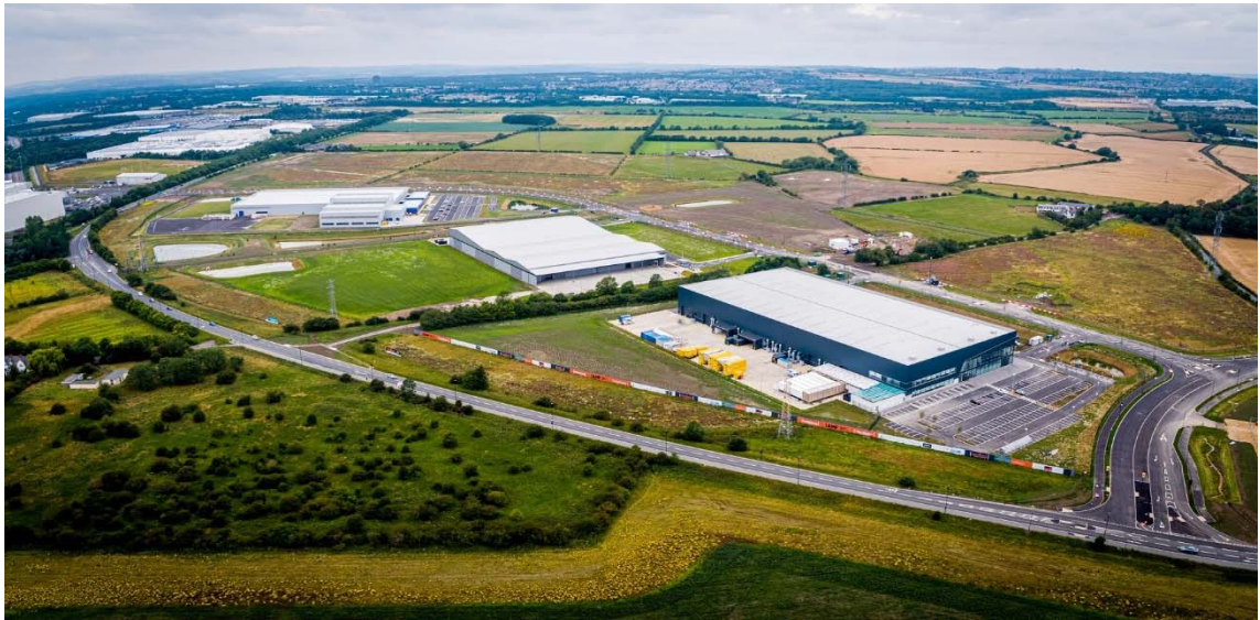
Figure 2.5 Photograph of the three industrial units looking westwards
