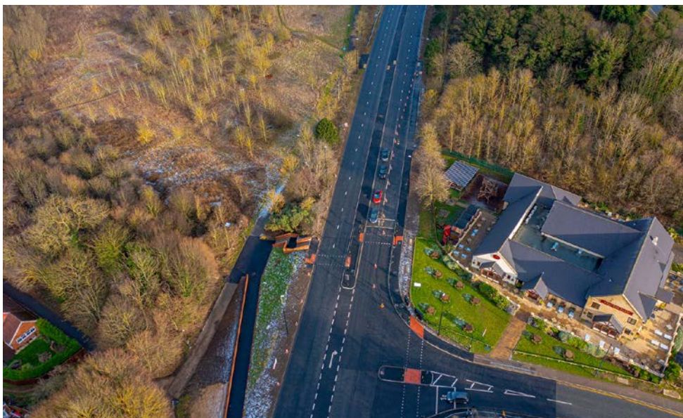
City Way Improvement Works, January 2023
