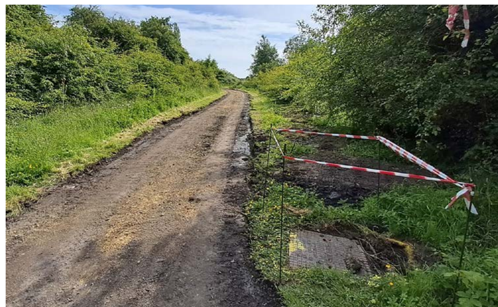
New multi-user route and wetland flushes preparation works, Success Railway
