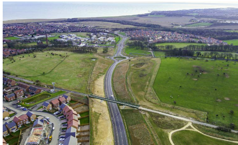
Completed RDLR and NMU, January 2024
