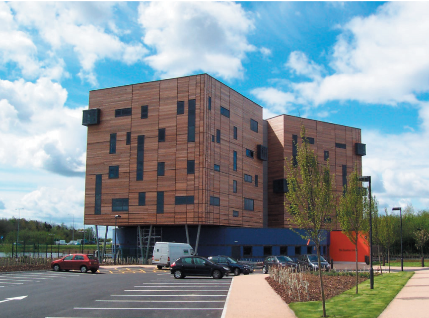
High quality managed office development, Quadrus Centre, Boldon Business Park.
