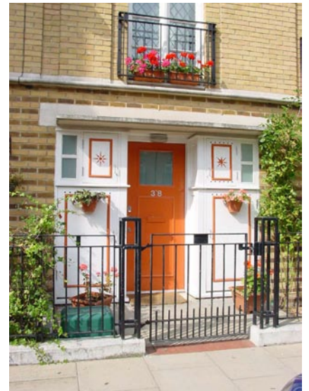
Active frontage with front garden, entrance and balcony
