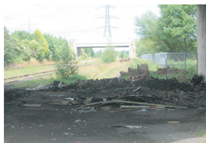
Dismantled railway line provides opportunity for pedestrian and cycle network
