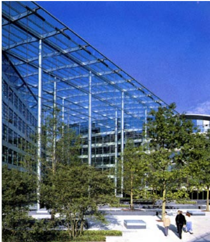
The use of glass to maximise natural solar gain
