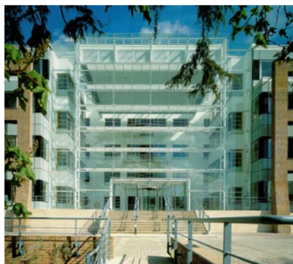
Successful integration of existing and new offices, Oxford Business Park
