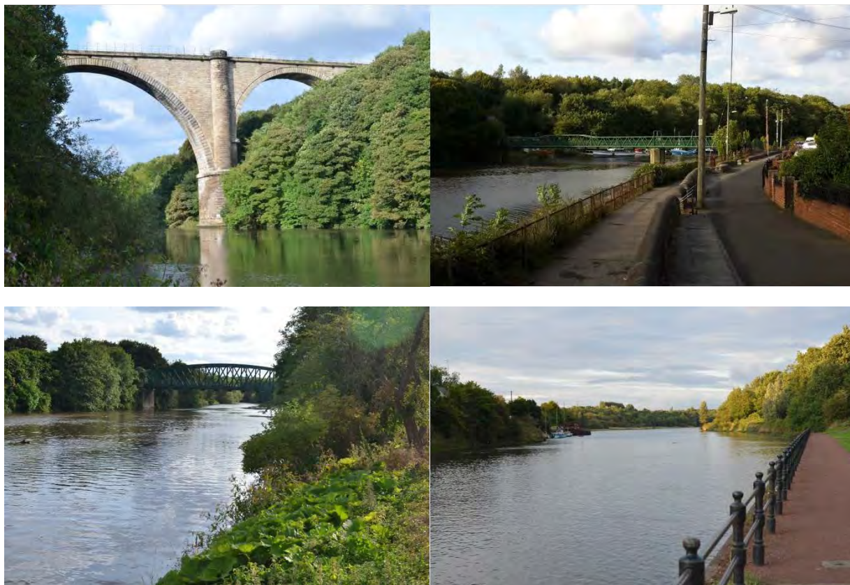
Clockwise from top left: grade II* listed Victoria Viaduct; footbridge at Cox Green; riverside at South Hylton; Penshaw Bridge at Fatfield.
