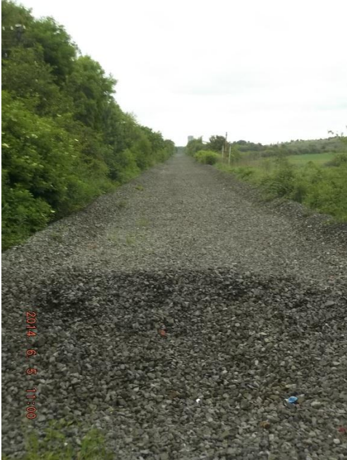
Figure B.19: View north along western boundary disused railway
