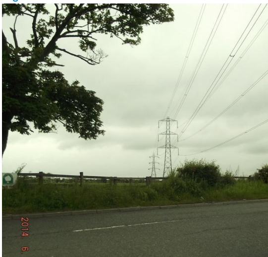
Figure B.11: View north from A1290
