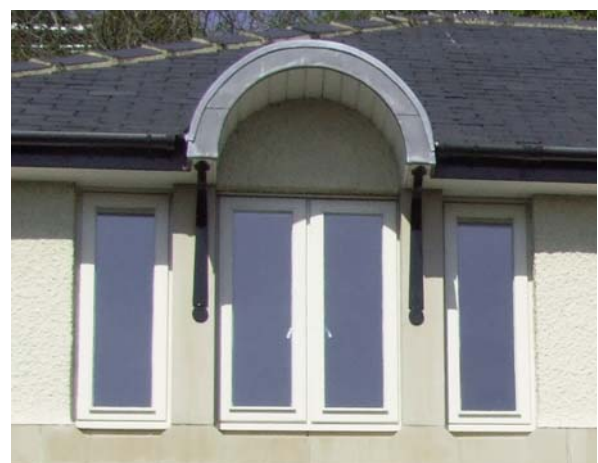
Arched window detailing in Thomas Hawksley Park.
