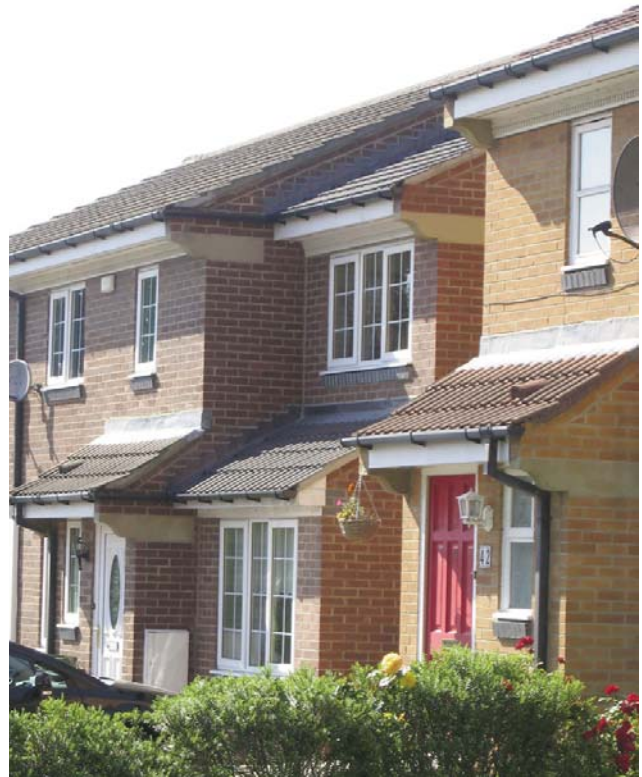
The examples of two storey side extensions show a set-back from the original front elevation. They are of an appropriate size in relation to the existing dwellings. The materials used match well with those of the original dwellings.
