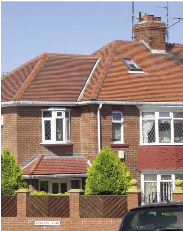
The examples of two storey side extensions show a set-back from the original front elevation. They are of an appropriate size in relation to the existing dwellings. The materials used match well with those of the original dwellings.
