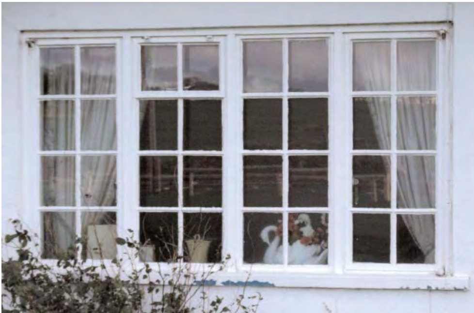
The photograph above shows the original window style to the front of the Bents Cottages. Under the provisions of the proposed Article 4(2) Direction original windows and doors will be required to be retained, or if beyond repair the style replicated, and encouraged to be reinstated where lost previously.
