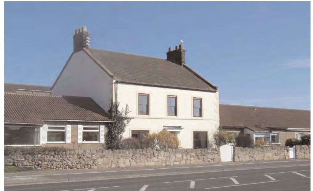
The bungalows built either side of South Bents Farmhouse detract considerably from the setting of this Listed Building. The materials used are particularly incongruous to the traditional character of the conservation area.
