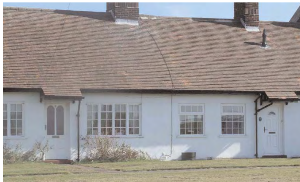
Changes to the window openings and windows to accommodate replacement PVC units have insensitively altered the historic form of the property to the right; the property to the left has retained its original appearance.
