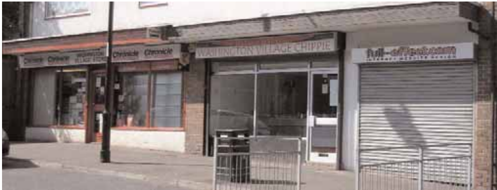
Above; poor signage and inappropriate security measures have a negative impact upon the area.
