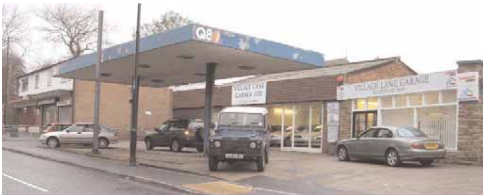
Above: modern shopfronts on Village Lane with unsympathetic signage and unattractive roller shutter security measures.
