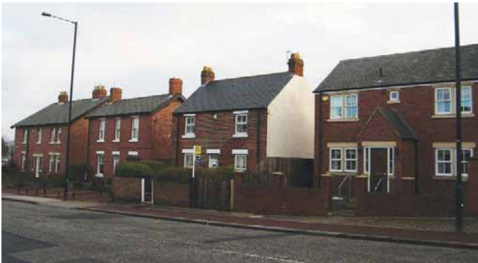
The recently built house to the far right of the picture respects and reinforces the building line, general form and materials of adjacent historic properties along this part of The Village unlike most 20th century development in the area. The ground floor fenestration does however appear a bit disproportionate when compared to adjacent historic buildings and the porch and boundary wall are not characteristic of the street.
