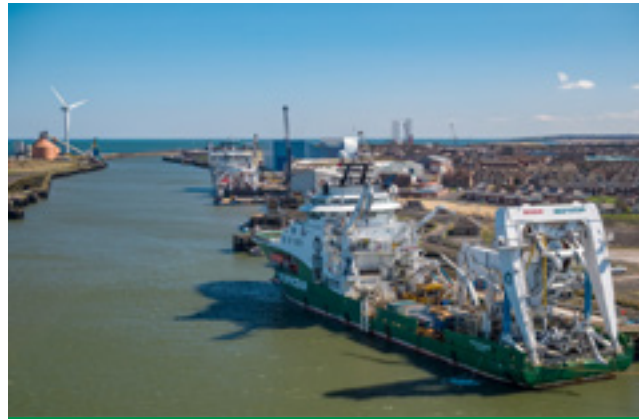
Port of Blyth in Northumberland – the second largest port in the region by turnover and a nationally significant offshore energy hub
