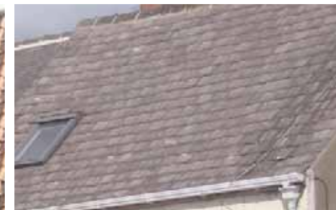
Welsh slate on Nesham Place
