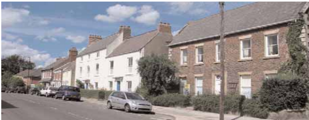
Nesham Place, the central street of the Nesham Place Conservation Area
