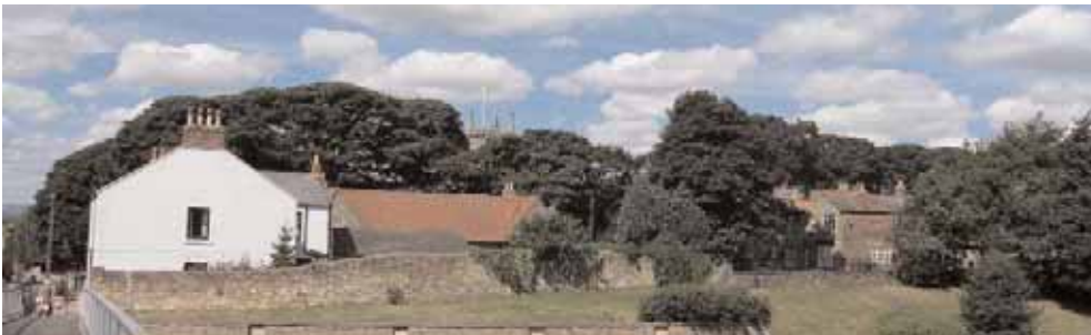
View into the St. Michael's Conservation Area from the footbridge to Nesham Place
