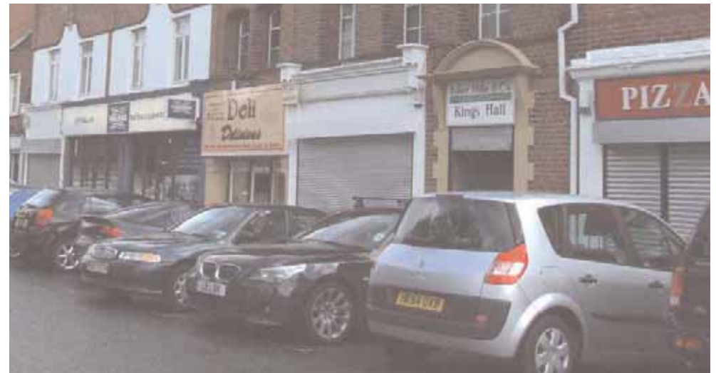
Above: modern shopfronts on Durham Road with unsympathetic signage and unattractive roller shutter security measures.
